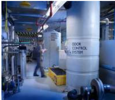
Treated Effluent Storage Tanks in Basement Equipment Room
